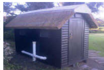
Refurbished restroom facilities
